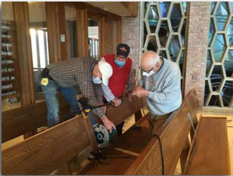
Members of the Facilities Ministry Team remove several pews in preparation for construction of a new Sound Booth.
